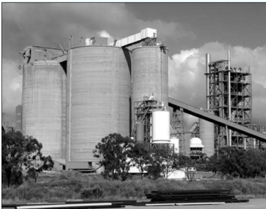
Cement Australia's plant at Fishermans Landing is working to reduce greenhouse gas emissions. qcl310105-1
